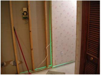
The laser lets me true up this stud that supports the existing drywall where it meets the door.
