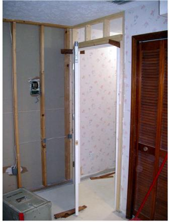
The next day I take on the door hang. Because the framing is true, it's way easier to hang the door. I balance the shims so the trim will be spaced from the hall walls the same on both sides. The laser level made sure the hinge side was plumb. Shimming up the door worked well to get everything where is is supposed to be.
