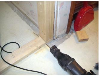
After a couple hours, I cut the bottom plate. It is anchored well, two screws per side, plus glue.
