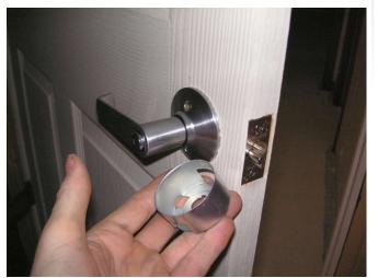
The lever would bind up in these thin doors, I left out this metal shield and they work fine.
