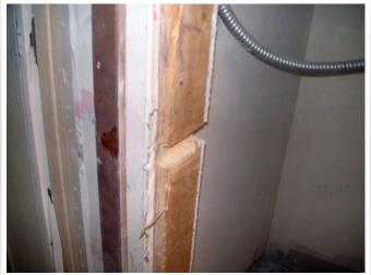
Then I cut the rest of the way with a Sawzall. I worked up and down from this notch.
