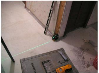
The Swanson 6-foot junk level is now only used as a straightedge to double check the laser.
