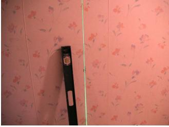
Here the laser is showing where the king stud goes on the perpendicular wall to the door.
