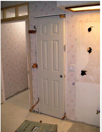
There were a lot of shims that needed readjusting as I pulled up the screws. The door seemed too wide, and I had to use a screw to open up the frame at the top. The top hinge got loose from hacking around the day before, so I replaced the screws with 1-1/4 drywall screws.
