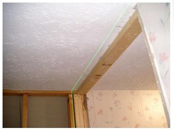
I get the top plate laid in with the help of the level. The king stud will support it at the wall.
