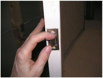
The Schlage latch is squarer than the mortise in the doors. A chisel squares off the corners.
