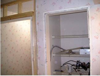
The door and trim goes easy, the drywall needed to come off around the periphery.
