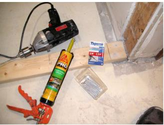
I put in the whole board for the bottom plate, using construction adhesive and Tapcon screws.
