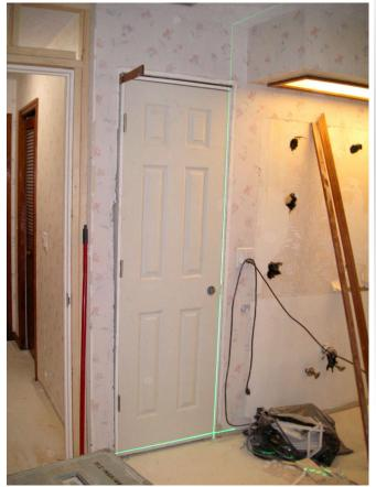
This is the headache I alluded to before. Since the hinge side of the door was all hacked up from the saw, I figured to "hang" the striker side. This all went sideways, and I just could not get the door hung right. I thought the stud where the striker jamb went was true. Wrong. There was no room for shims on both sides.
