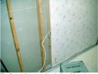
The Romex becomes detached, and I put in a new stud drilled and with a nail plate.
