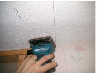
I figured to get ahead of things and sand the ceiling flat where I will have to drywall tape.
