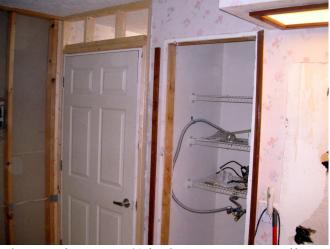
The opening was 1/4-inch too narrow. I nail a guide strip up for the circular saw.
