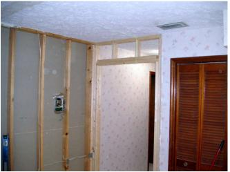
In go the jack studs, the header, and a couple cripple studs.
