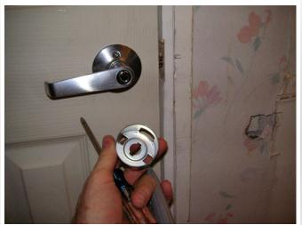
Flip the levers around, and leave out the same shield so the levers don't bind. This will be replaced with a 'passage' style, no need to lock.
