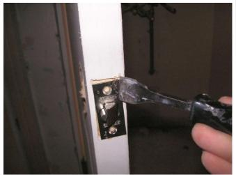
When the door closed OK, I put in the same Schlage latch plate, with a little help from a chisel to square off the mortise corners.
