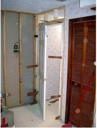
With the laser on, I get the shims perfect, screw in the frame then put a long screw in the hinges. Once the hinge side is true, I can set up the gap on the striker side with those shims. The door sprung open an inch, these Jen-Weld doors are cheap, you need a little more skill, and most of all, patience, to get them hung, keep watching.
