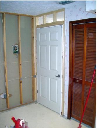
The door is in. I like solid-core doors because they block noise way better, and because their weight means you can just swing them and they have the momentum to close and latch. That thing on the wall is the back of an intercom. I suspect I will tear off all the drywall on the right side wall. I have medicine cabinets there.
