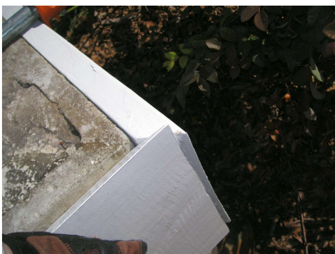
The board is a little long, I trimmed it and re-painted the raw edge.
