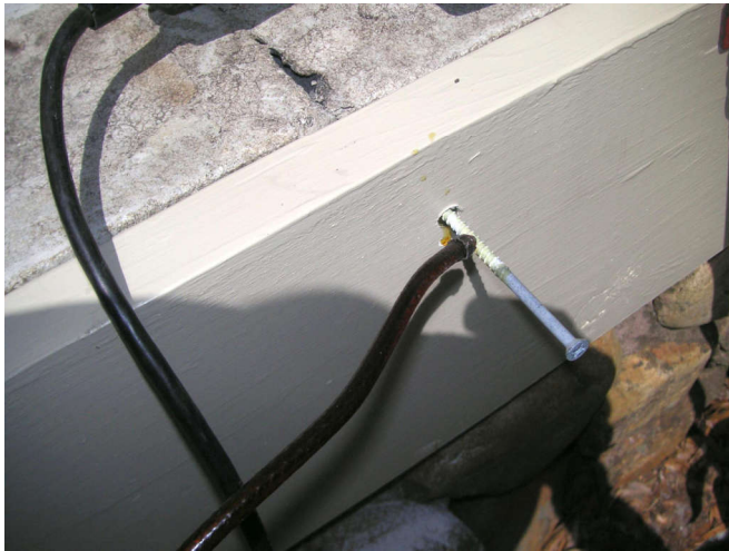
I learned to put some 15W50 motor oil on the screws to get them to drive all the way in.
