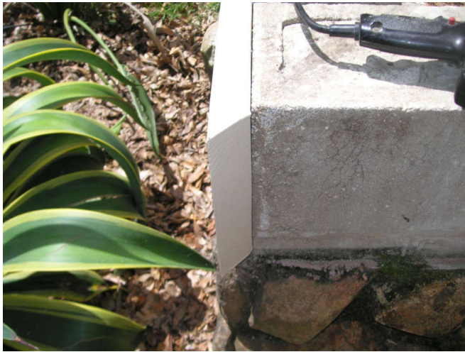
That last screw drove all the way in, and pulled the board flat against the cinder block.
