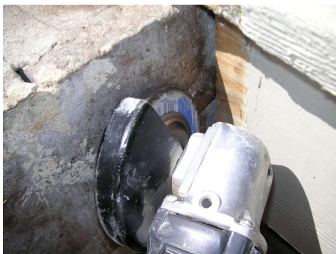
A right-angle grinder cut out the rebar.
