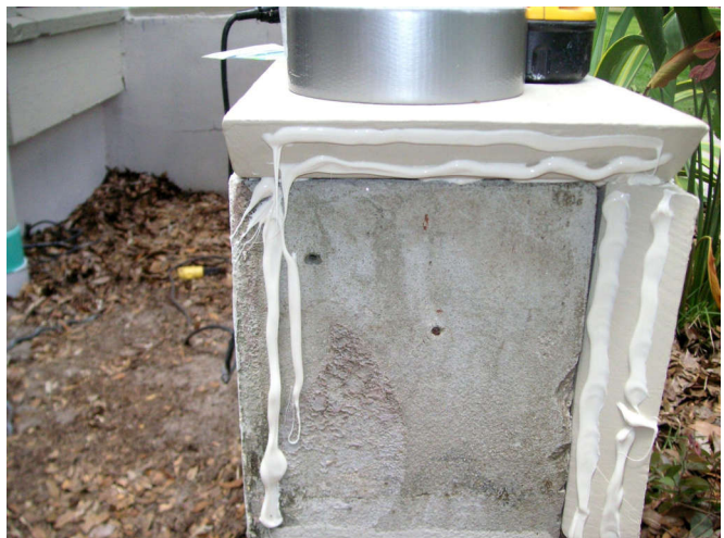
I caulk up the end cap area with enough silicone to squeeze out and make a good seal.
