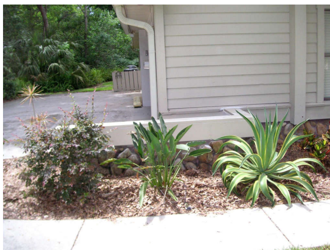
A front view of the wall from a distance.
