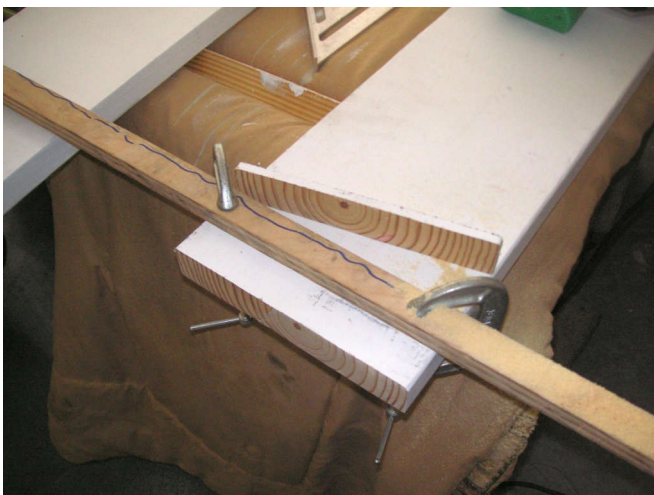
I set up in the garage, and used to the Hitachi saw to cut about a 1/4" from the board. This was too much, I might have got away with an 1/8". Short is better, you can fill with caulk.
