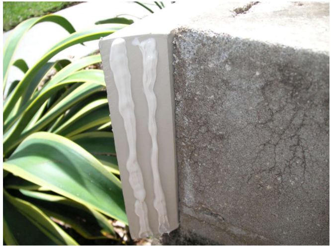
I lay in two thick beads at the corner.
