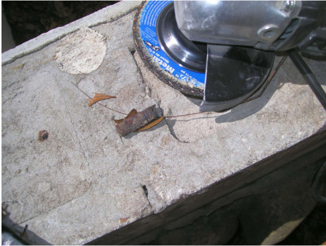
This meant the original lumber never fit right.
