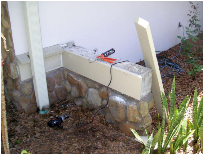
Four screws hold the side board on.
