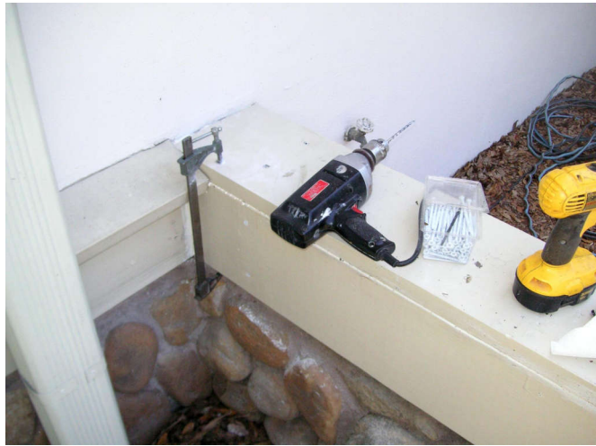
Another clamp pinned the top piece while I drilled for the screws.
