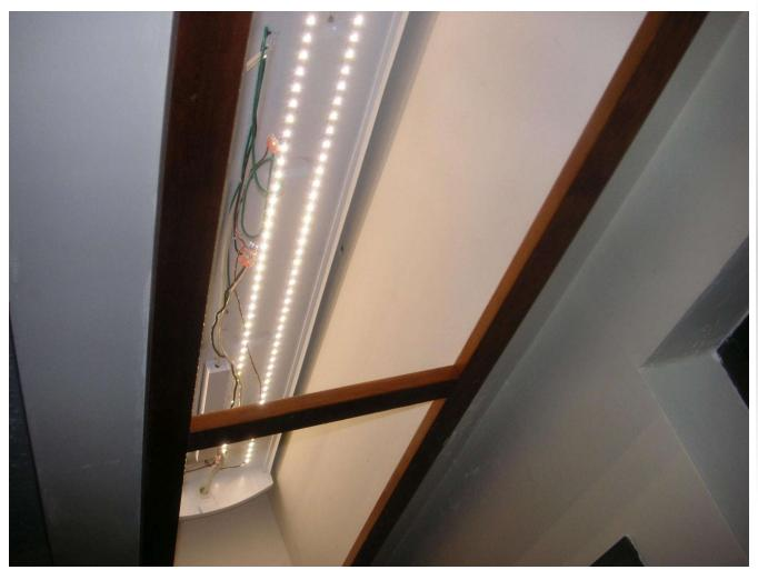
My house was built around 1986, when soffits for the baths and kitchens were all the rage. The bathroom soffits hold 4-foot florescent fixtures. Some were flickering, some were buzzing, the master bath lamp was doing both. Rather than try to put in new bulbs, new starters, or new ballasts, I took the opportunity to replace the whole fixture with ultra-bright daylight color temperature LED lamps.
