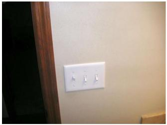
Here is the new switches and cover plate. Lowes sells switches without a surround bezel around the lever. Home Depot sells these switches, that do have the little bezel around the lever that sticks through the holes in the plate. I am not yet sure which I like better. The switches without bezels have a wider lever, which is nice.
